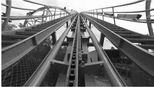
Figure 5. Above: Frame number 839 in [3], unedited. Below: The undistorted frame.
