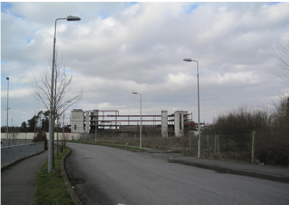
Figure 3.7: Downshire Centre Development, Partially constructed ‘Edenderry Plaza Hotel’.
