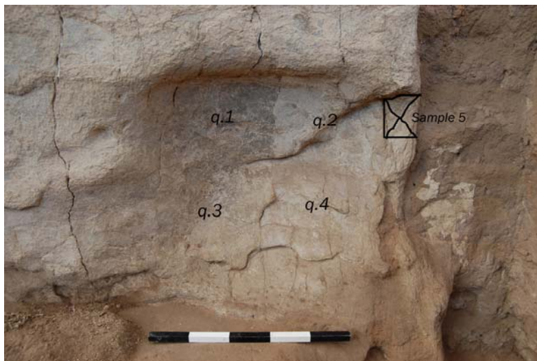
Figure 175: Building 5, F.245 in south wall (F.244). Photo Kelly Caldwell
