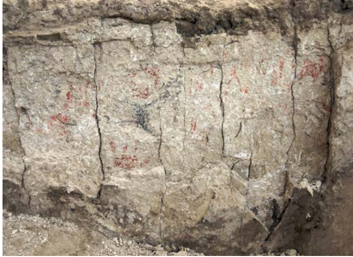
Figure 176: Wall painting in Building 55
